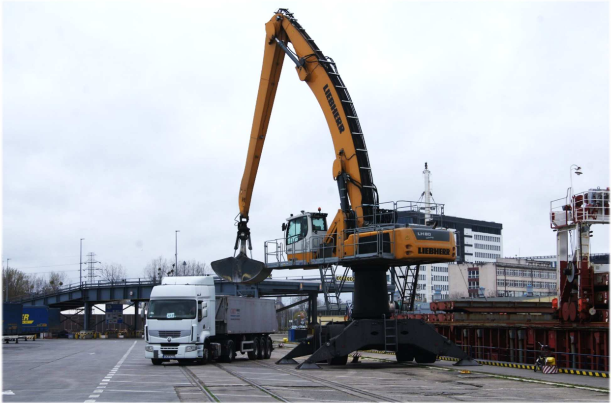
phot. Liebherr mobile cranes LH 80 on Czeskie Quay.
